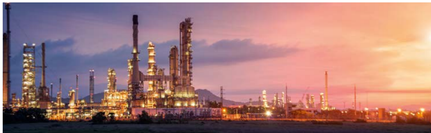
KLINGER UK provides a wide range of on-site services for refineries
