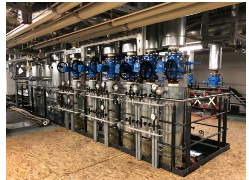
A row of DN 150 KLINGER Ballostar KHI ball valves installed at Erdwärme Grünwald
