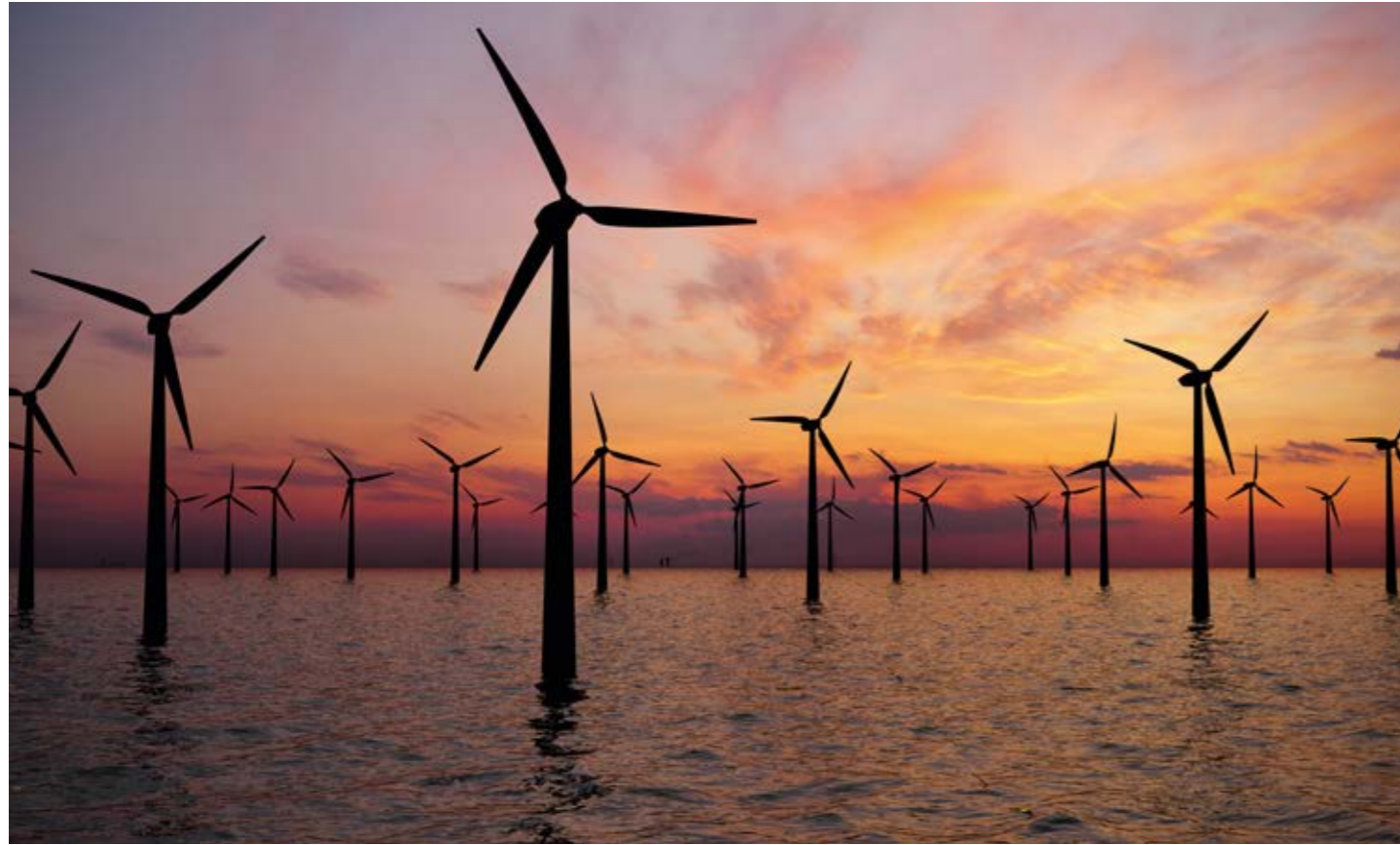
The slip rings supplied by KLINGER UK play an important role in ensuring the smooth operation of wind turbines
