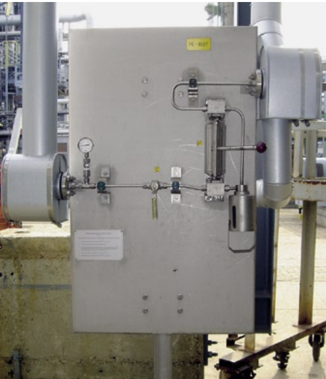
AB-cocks for pressure transducer stations.
