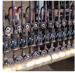
leaking or just plugged, highlighting the need for the steam trap survey conducted by the Dutch KLINGER subsidiary. These inspections of the three assets were the starting point for a major corrective maintenance program aimed at replacing and modernizing the existing steam traps.
