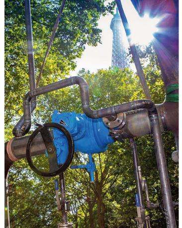
The KHSVI VVS DBB with mechanical AUMA actuator is already seeing active use in the district heating network of Paris.
