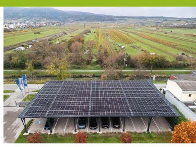
The carport's 642 square meters of PV-equipped roofing generates 113 kilowatts of electricity.
